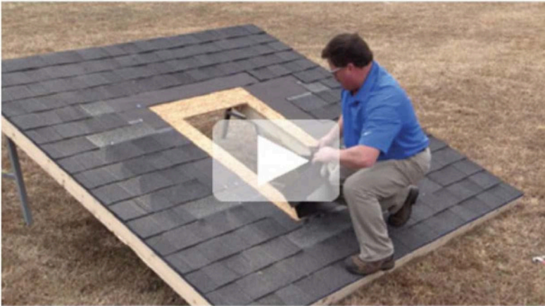
VELUX Install Video: Replacing Deck-Mount Skylights
