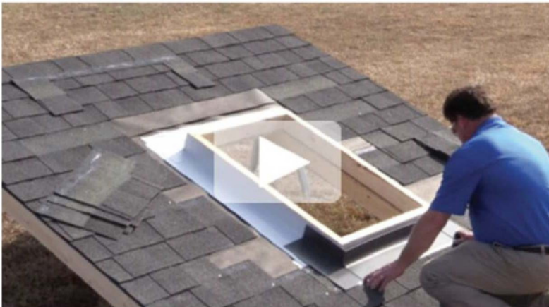
VELUX Install Video: Replacing Curb-Mount Skylights
